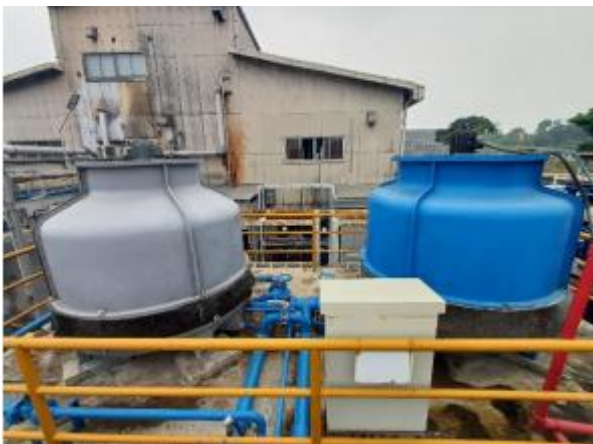
Gambar 3. Tipe induced draft cooling tower
